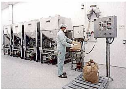
Container feeding stations and operator-controlled manual additions
